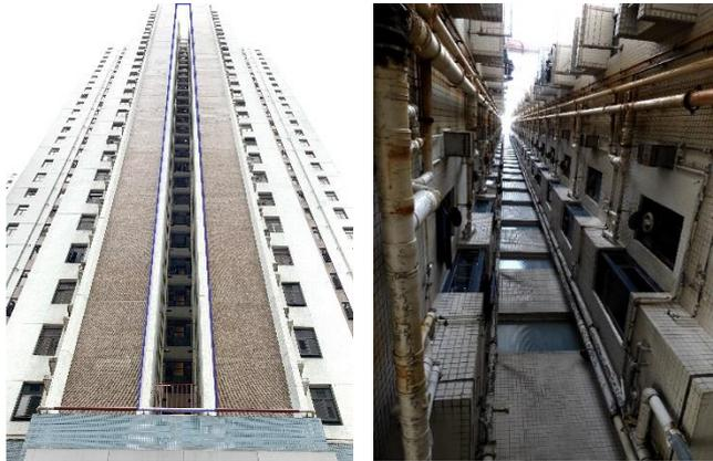
Window at habitable area facing a four-side enclosed yard (non-compliant)
