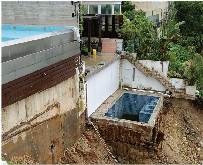
Figure 8: Example of “serious UBWs” (last year’s rainstorm revealed some large-scale UBWs in certain houses, such as the unauthorised swimming pool shown in the photo below, with landslides occurring on the surrounding slope)
