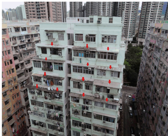
Figures 6 and 7: “Street shadow building” (the arrows in red are pointing at UBWs, which are canopies erected at places that have been set back)
