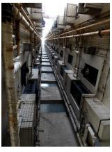
Window at habitable area facing a four-side enclosed yard (non-compliant)
