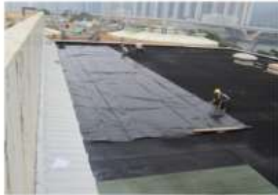
Proper installation, protection and upkeep of waterproofing layer on roof/podium
