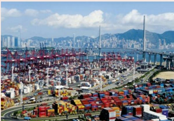
In 2016, Hong Kong's harbour handled 19.8 million TEUs (20-foot equivalent units) of containers, making it one of the world's busiest container ports. The nine container terminals at Kwai Chung-Tsing Yi are managed by five operators. They cover 279 hectares and provide 24 berths with a frontage of 7 694 metres. The water depth at the Kwai Chung-Tsing Yi basin is 15.5 metres.
