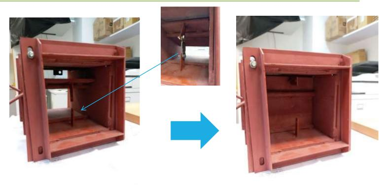
A fire damper is in open position under normal condition, and will be closed during fire incident to prevent the spread of fire
