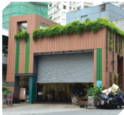
Current Refuse Collection Point in urban district
