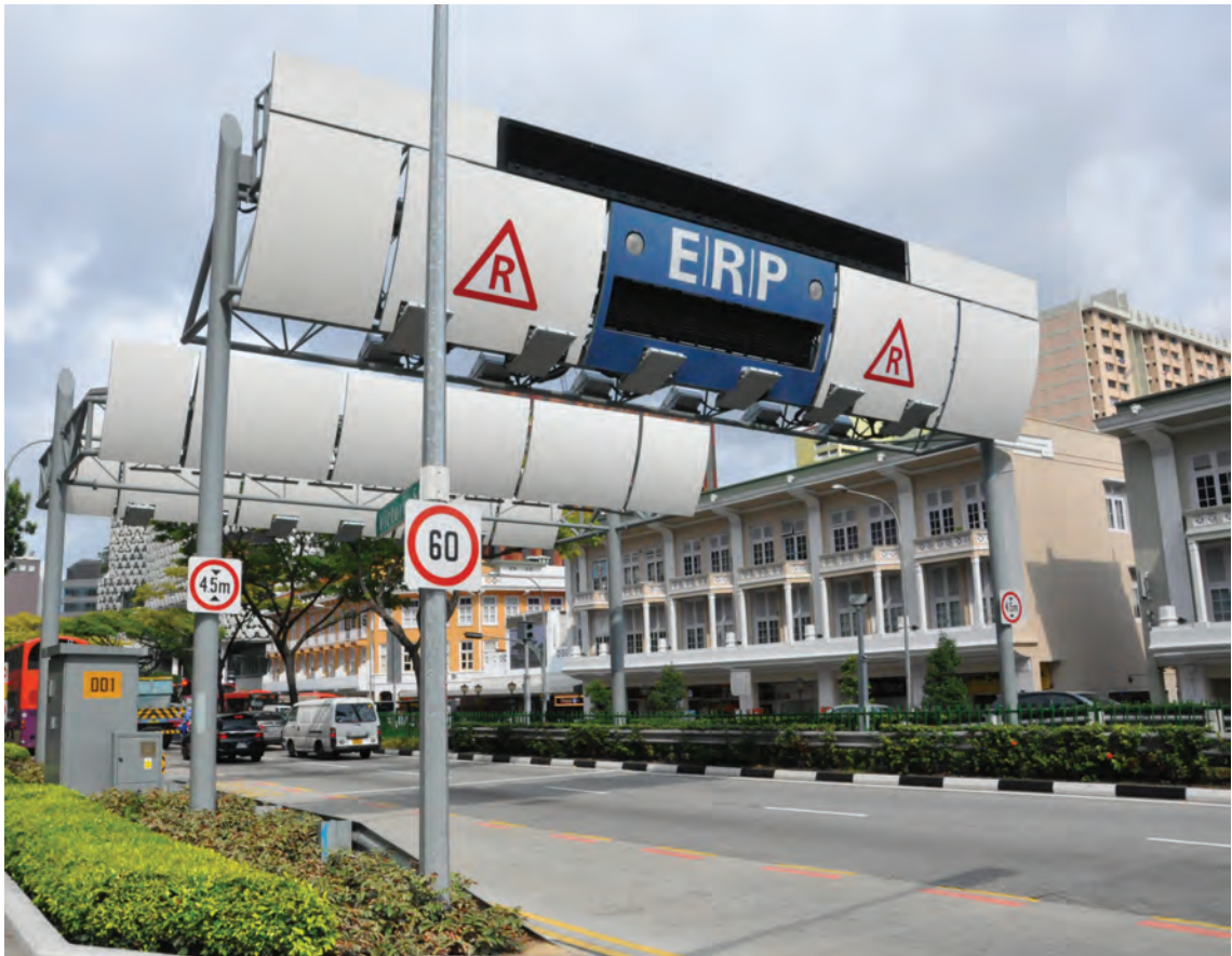
Figure 3.2A – A typical ERP gantry
