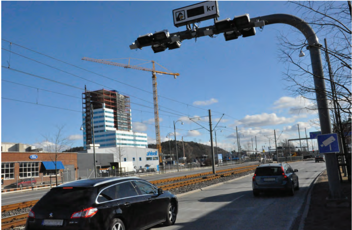
Figure 3.8 – Roadside ERP gantry in the Gothenburg Scheme
