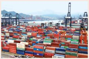
In 2013, Hong Kong's harbour handled 22.35 million TEUs (20-foot equivalent units) of containers, making it one of the world's busiest container ports. The nine container terminals at Kwai Chung-Tsing Yi are managed by five operators. They cover 279 hectares and provide 24 berths with a frontage of 7 694 metres. The water depth at the Kwai Chung-Tsing Yi basin is 15.5 metres.
