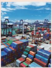
In 2010, Hong Kong harbour handled 23.7 million TEUs (20-foot equivalent units) of containers, making it one of the world's busiest container ports. The nine container terminals at Kwai Chung-Tsing Yi are managed by five operators. It covers 279 hectares and provides 24 berths with a frontage of 7 694
